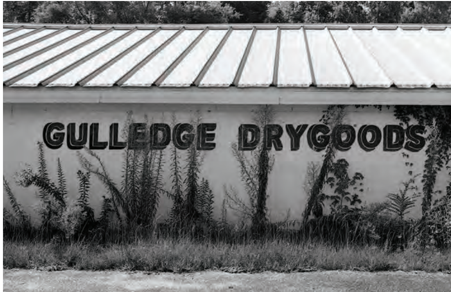
Former Gullede Drygoods, Clayton, AL (Photo by Emily Rena Williams)
